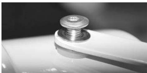
Detail of the mounting of the bracket with bolt, washer and silicon washer.
